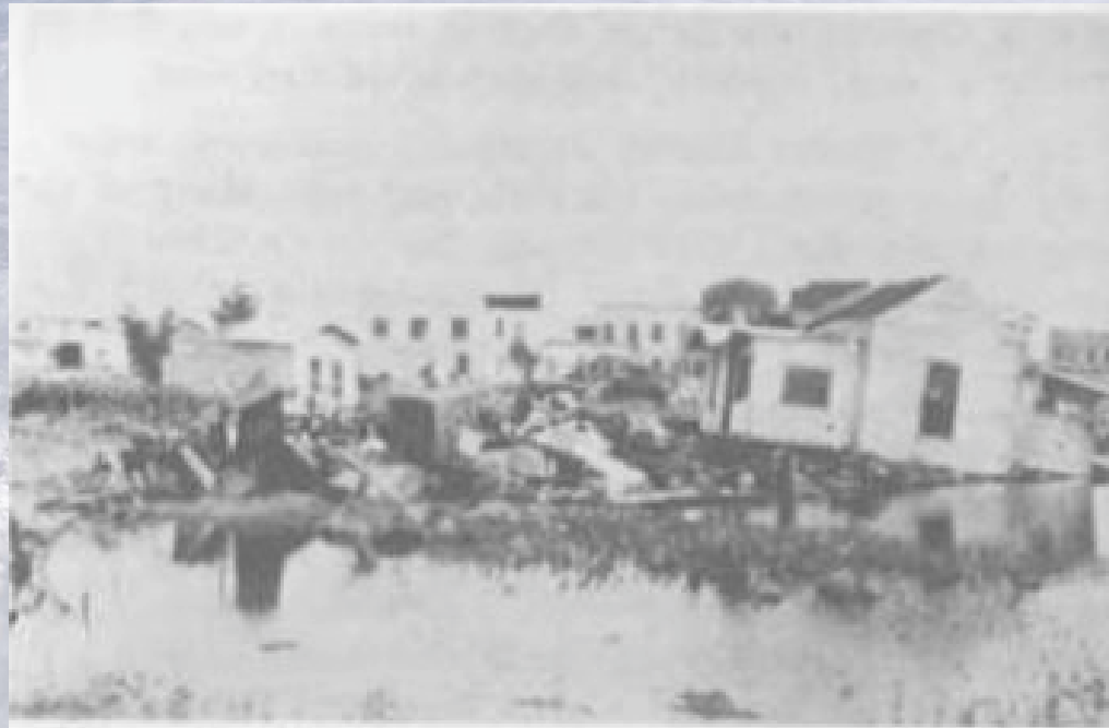
Belle Glade: Wreckage of Ford garage. Borer building (left); Pioneer building (right).
